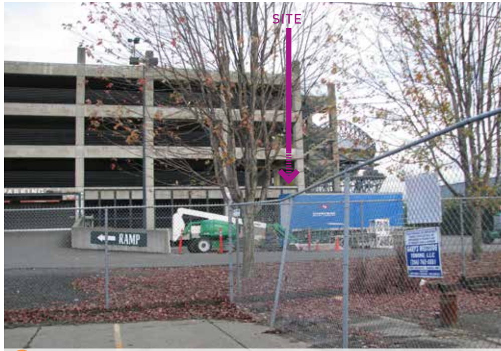
1 VIEW NORTH FROM S. MASSACHUSETTS ST.
