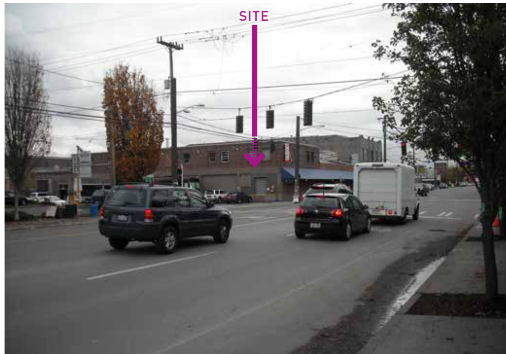
4 VIEW SOUTH ON 1ST AVE S.
