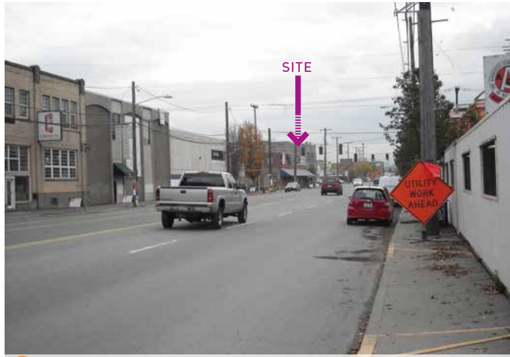
1 VIEW SOUTH ON 1ST AVE S.
